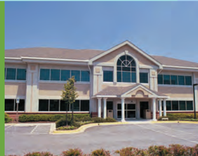
Dunkirk Medical Building
